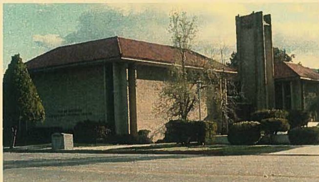
1972 to present: Glendora Public Library and Cultural Center
